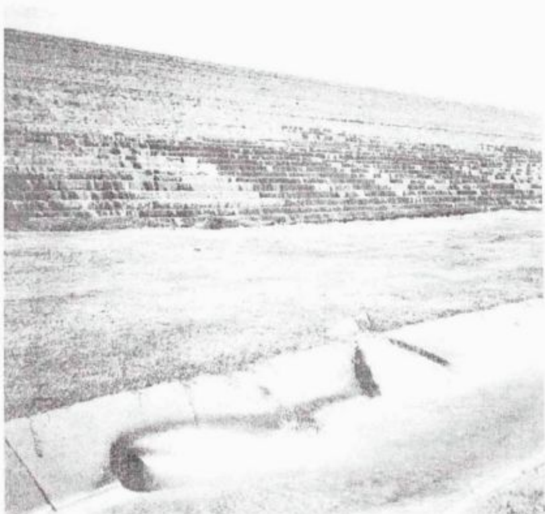
Figure 4.6. Photograph of the old fly ash dam at Kriel Power Station, showing the wet fringe around the bottom portion of the dam and cut-off drain with penstocks decanting water.
