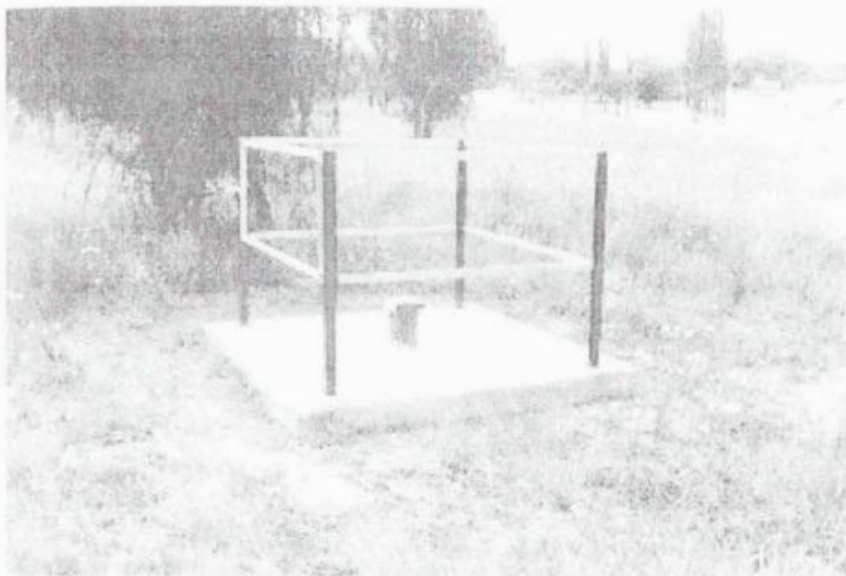
Figure E.3. Example of a secure structure around a monitoring borehole at Komati Power Station.
